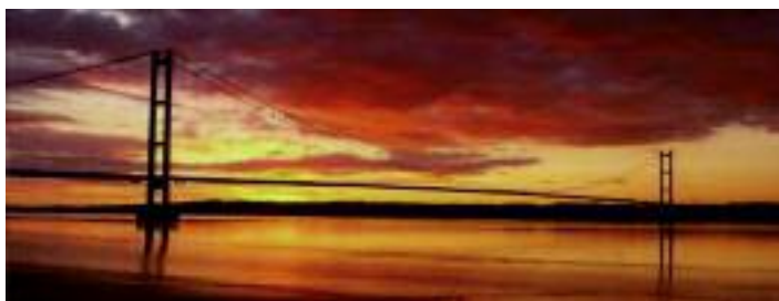
Le Humber Bridge, Kingston Upon Hull
